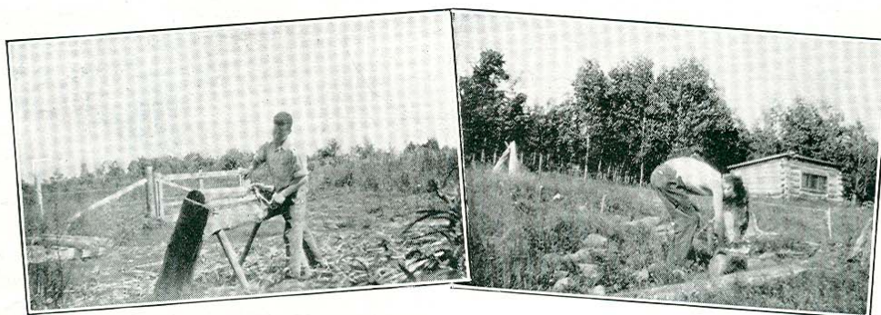
Cedar was used in building temples thousands of years ago; this boy builds a cabin in Happy Land in 1928 with the same fragrant durable wood—here he is removing the bark with a drawknife.
